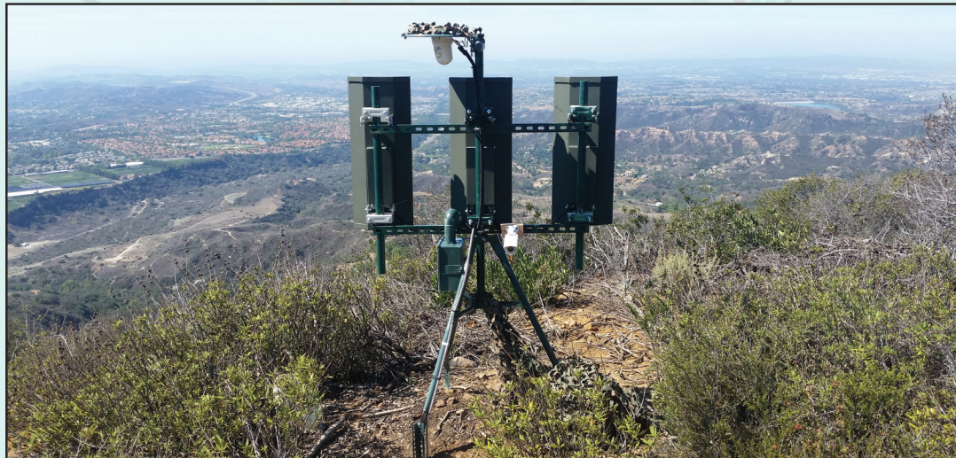
AE6XE Orange County California 3 node installation
